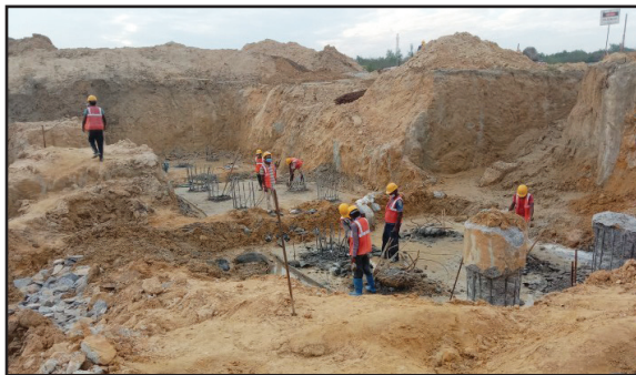
Chipping Work in Progress at CGF (Simplex) at TFL Talcher
